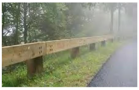
Steel-backed wood guardrail—front
