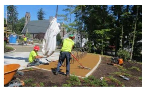
StaLok aggregate—high traffic/slope
