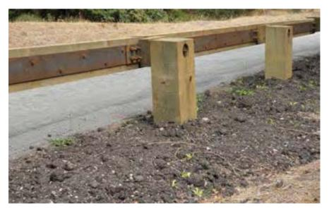
Steel-backed wood guardrail—back
