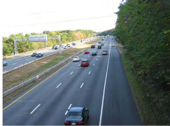
Route I-95 /128 south of Kendrick Street
