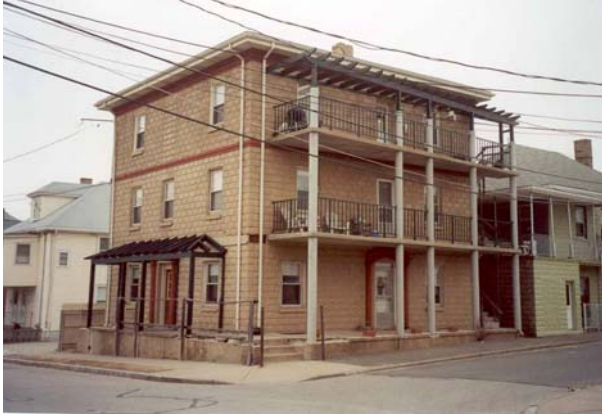
78 Hawthorne Street – Feb. 2001
