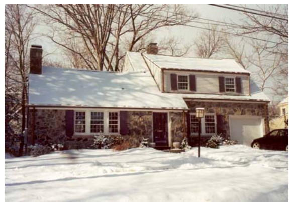
24 Nickerson Road – Feb. 2001
